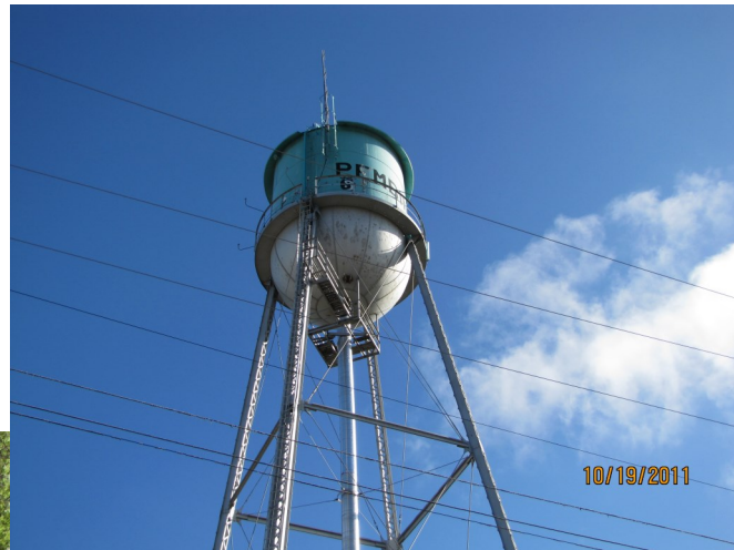
Pembina water tower—replace main pipe.
