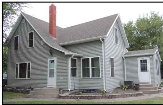
After: New windows, doors, siding and shingles
