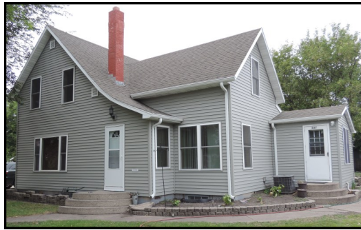
After: New windows, doors, siding and shingles
